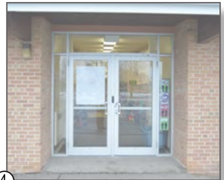
④ ALUMINUM DOORS & ALUMINUM STOREFRONT
